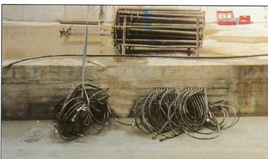
◀ View after completion.
