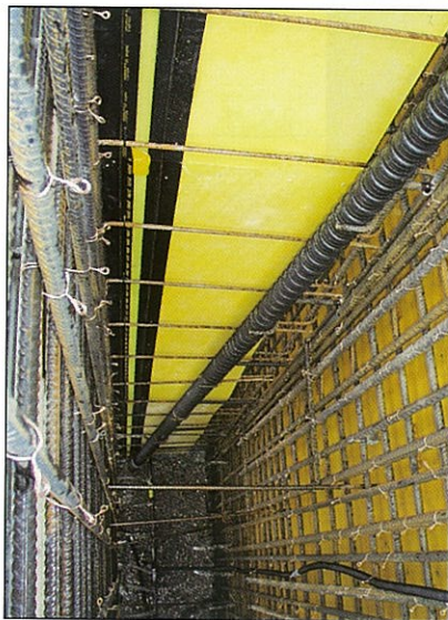
Widened RASCOTec ▶ crack-inducing unit between reinforcement.
