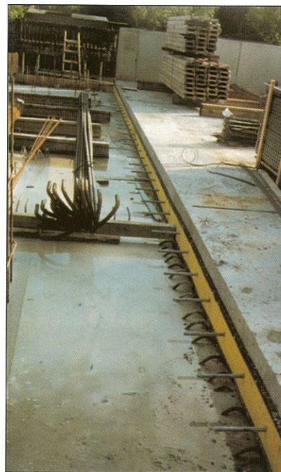
◀ RASCOtec expansion joint units can also be incorporated in movement joints designed to transmit transverse loads.
