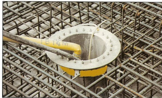
◀ Sealing of a groundwater relief pipe in a ground slab.
