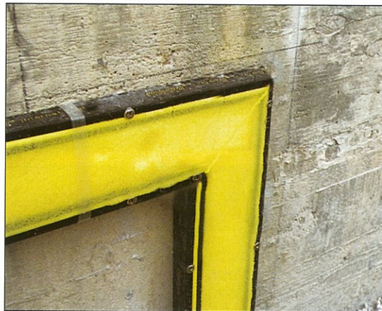
◀ Angle formation of RASCOtec expansion joint unit.
