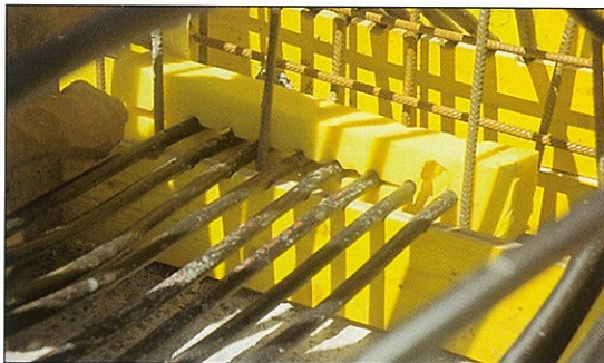
▲ Where injection collars are directly cast in, these are drilled into and grouted after concreting.
