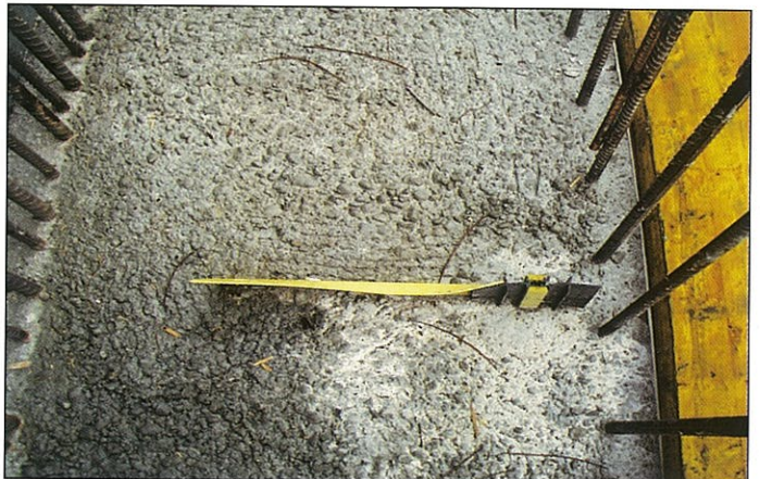
▼ Widened RASCOTec crack-inducing unit after concreting.
