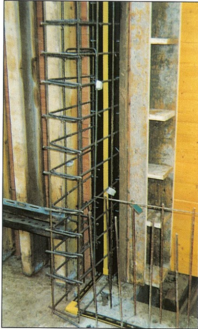
RASCOTec ▶ crack-inducing unit incorporated in wall formwork.
